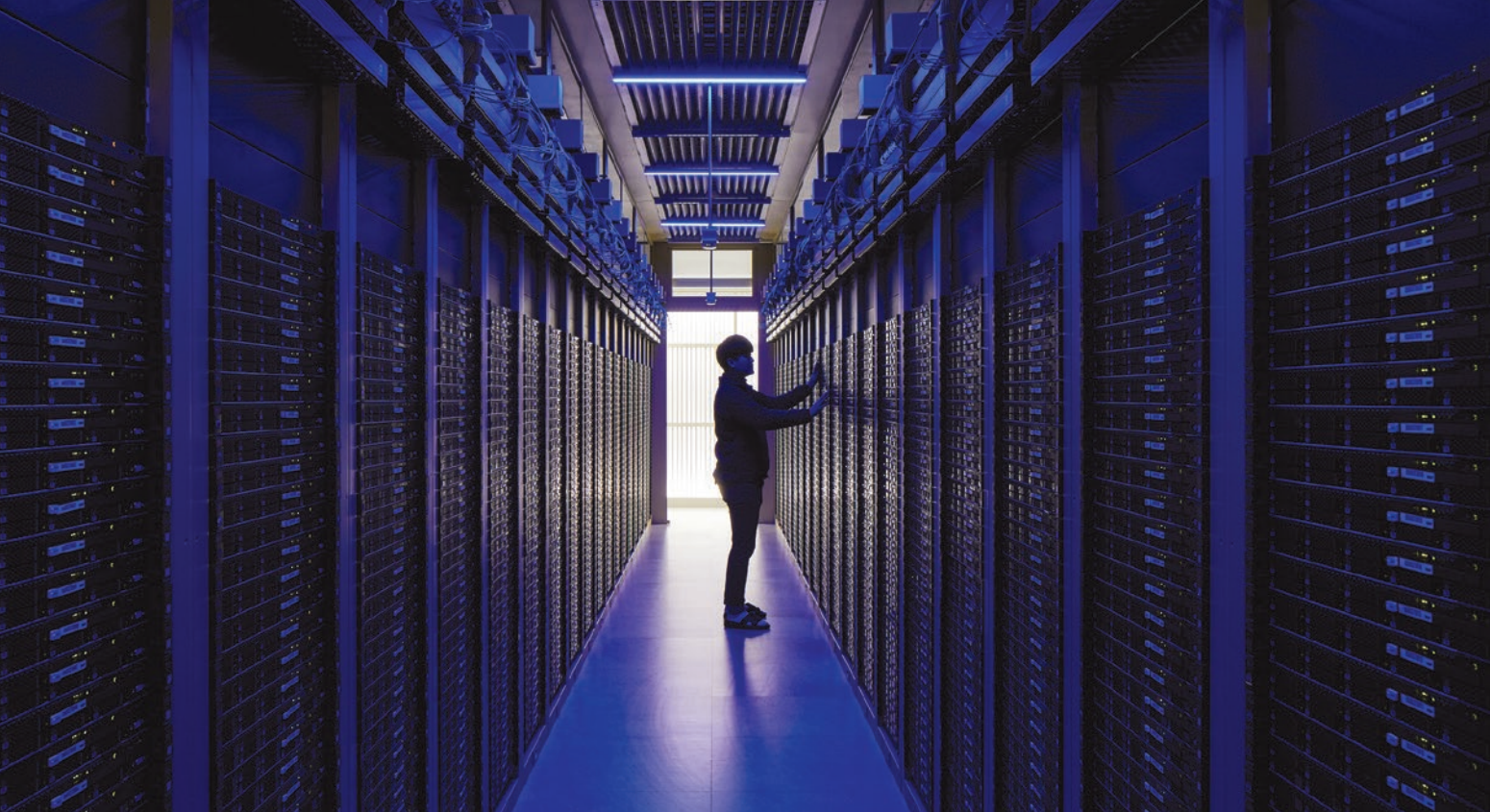
Data Center Gak
